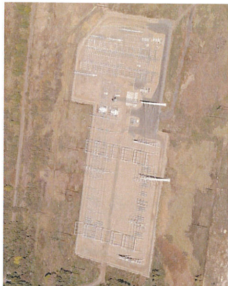
Midvalley Substation. 345 kV to 138 kV
